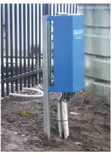
Antennae cables in conduit linked to **CALCLEAR** control box. Brookvale Oval, NSW
