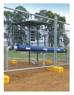
Prewound pipes installed above ground for water supply. Liverpool Plains Council, NSW.
