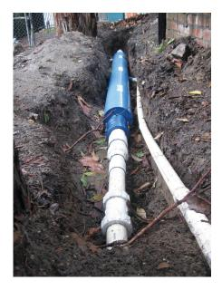
**CALCLEAR** prewound pipe with protective outer pipe being installed below ground.
